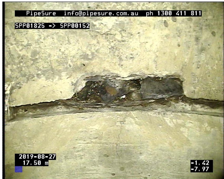
Photo: 1_3A, Media No:: 280819_1, 00:05:35 17.5m, Breaking, some pieces are missing, length of break: 100mm, at 12 o'clock
