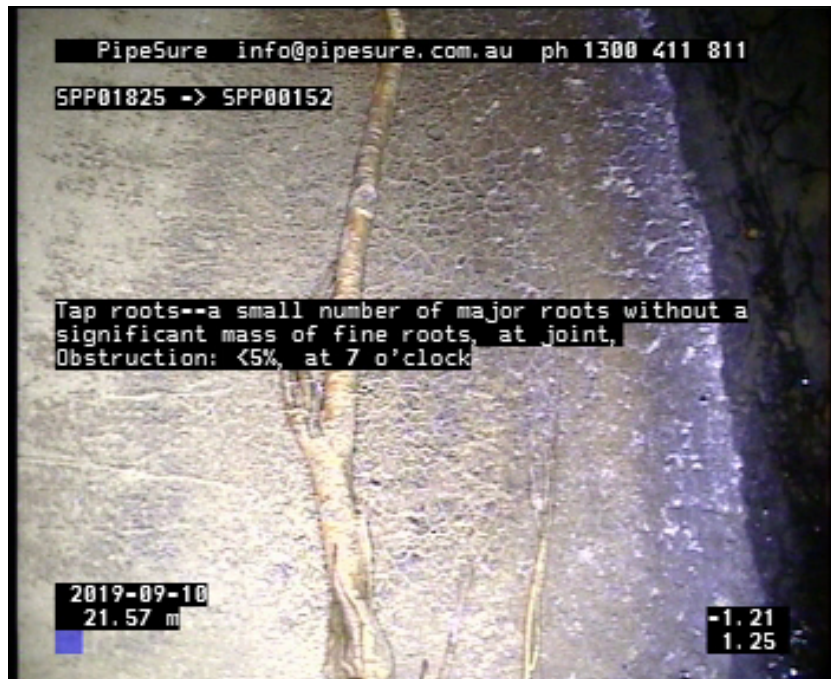
Photo: 1_9A, Media No:: 100919_1, 00:07:24 21.57m, Tap roots--a small number of major roots without a significant mass of fine roots, at joint, Obstruction: <5%, at 7 o'clock
