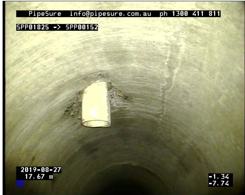
Photo: 1_4A, Media No:: 280819_1, 00:05:50 17.67m, Intruding connection, magnitude of intrusion: 5-20%, at 11 o'clock, 100mm pvc / 100mm pvc
