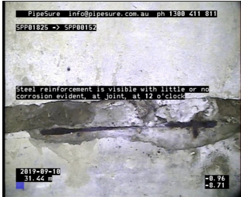
Photo: 1_14A, Media No:: 100919_1, 00:10:56 31.44m, Steel reinforcement is visible with little or no corrosion evident, at joint, at 12 o'clock
