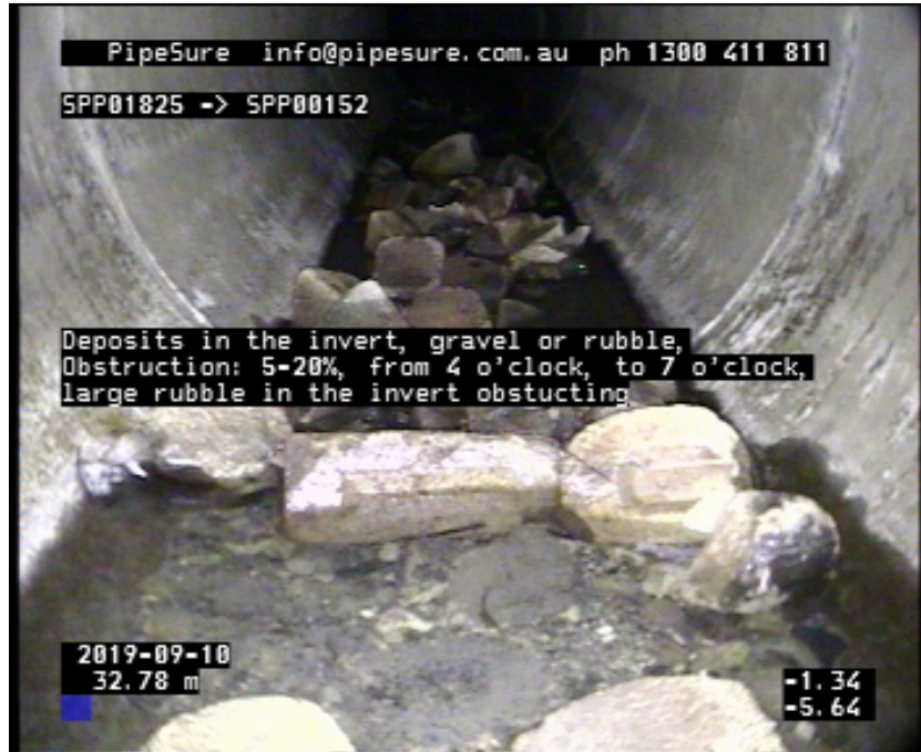
Photo: 1_15B, Media No.: 100919_1, 00:11:33 32.78m, Deposits in the invert, gravel or rubble, Obstruction: 5-20%, from 4 o'clock, to 7 o'clock, large rubble in the invert obstructing / large rubble in the invert obstructing
