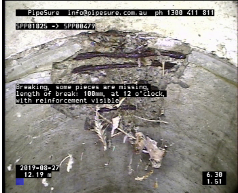
Photo: 3_9A, Media No:: 280819_1, 00:06:56 12.19m, Breaking, some pieces are missing, length of break: 100mm, at 12 o'clock, with reinforcement visible / with reinforcement visible
