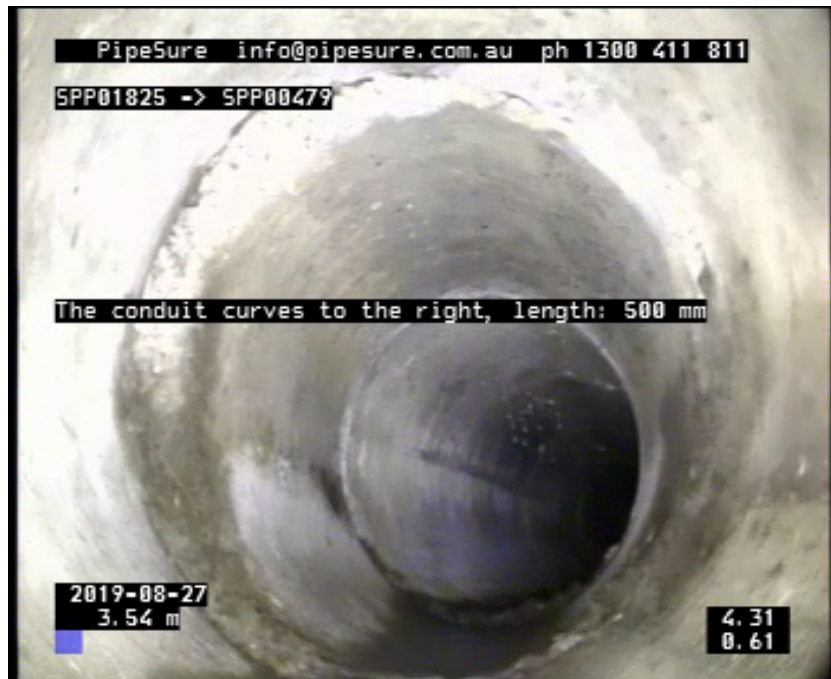
Photo: 3_5A, Media No:: 280819_1, 00:02:22 3.54m, The conduit curves to the right, length: 500 mm
