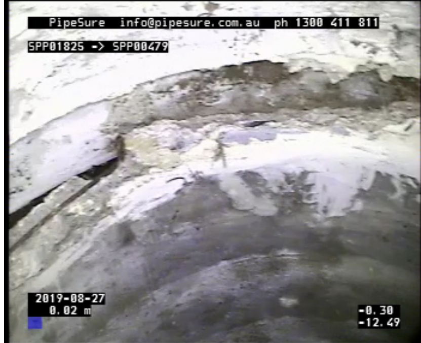
Photo: 3_2A, Media No:: 280819_1, 00:00:39 0.02m, Joint displaced longitudinally, longitudinal displacement: >30mm, at 11 o'clock
