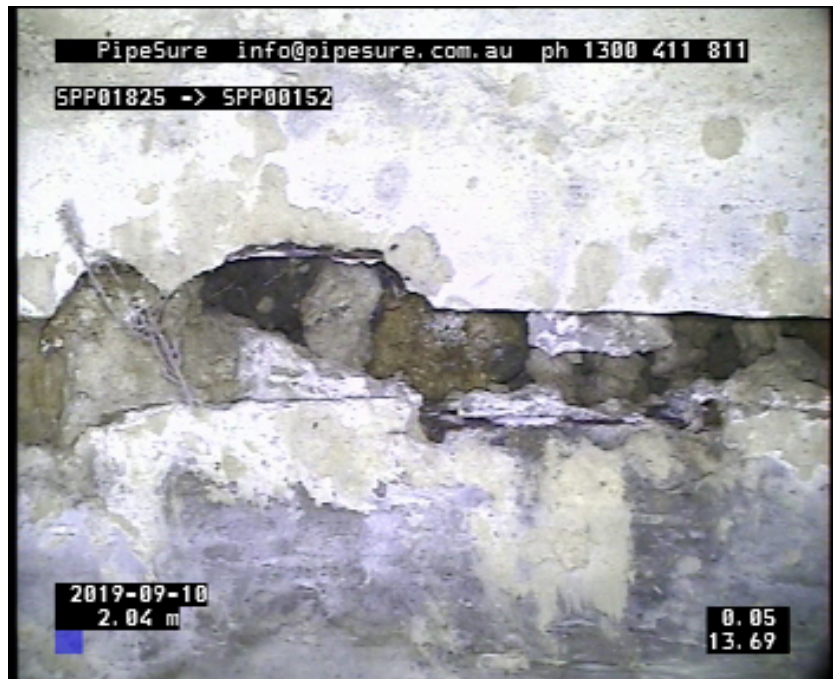
Photo: 1_4A, Media No:: 100919_1, 00:01:32 2.04m, Missing mortar, depth less or equal to 15 mm, at joint, at 12 o'clock
