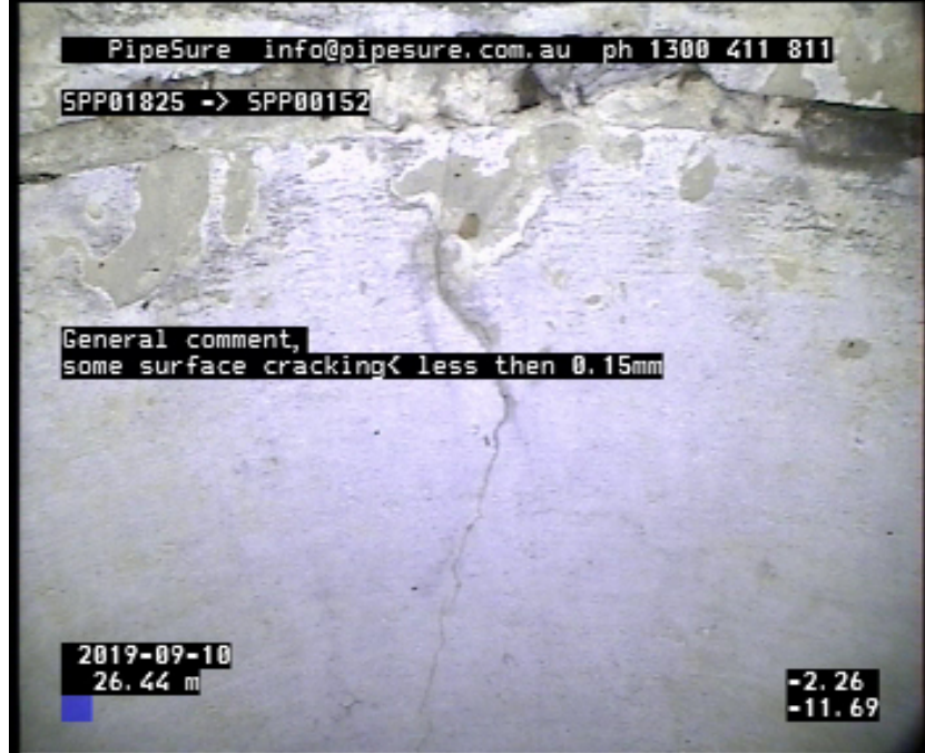
Photo: 1_12A, Media No:: 100919_1, 00:09:06 26.44m, General comment, some surface cracking< less then 0.15mm / some surface cracking< less then 0.15mm
