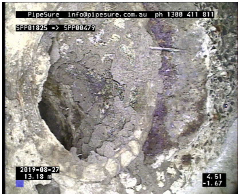
Photo: 3_10A, Media No:: 280819_1, 00:07:45 13.18m, Connection, poor workmanship, connection appears to be open, height: 225 mm, width: 0 mm, at 8 o'clock
