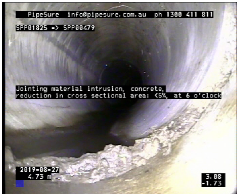
Photo: 3_7A, Media No:: 280819_1, 00:03:08 4.72m, Jointing material intrusion, concrete, reduction in cross sectional area: <5%, at 6 o'clock
