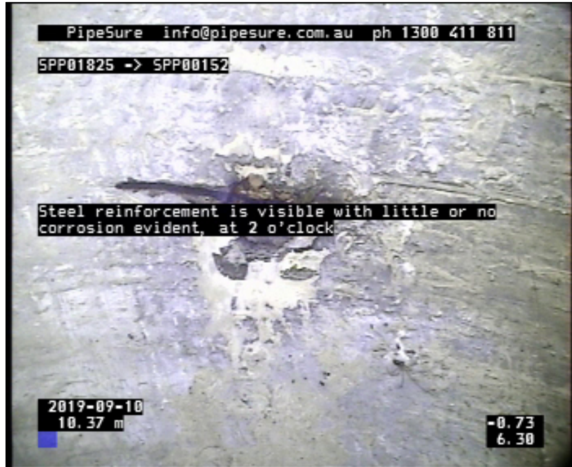
Photo: 1_7A, Media No:: 100919_1, 00:04:13 10.37m, Steel reinforcement is visible with little or no corrosion evident, at 2 o'clock
