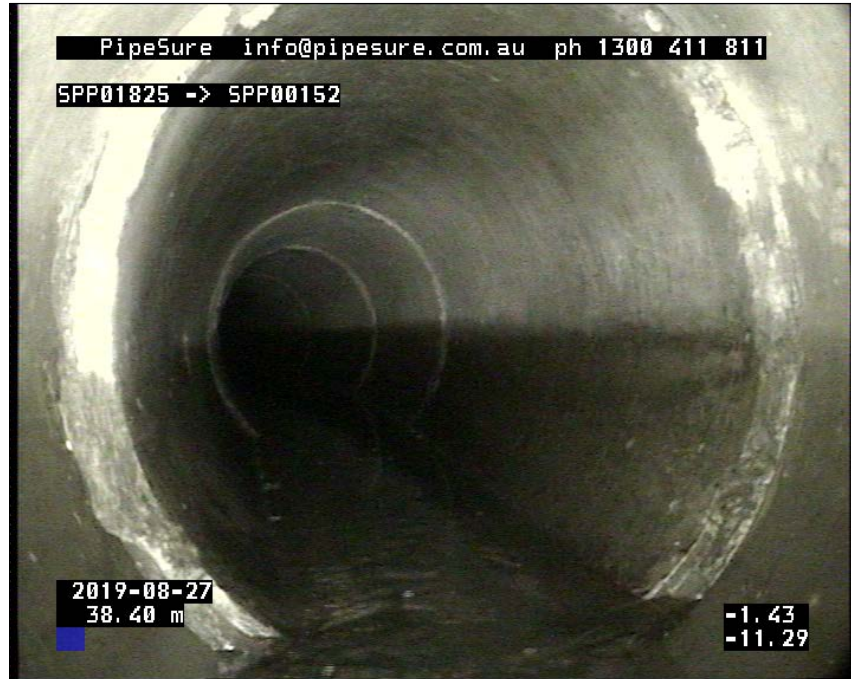
Photo: 1_6B, Media No:: 280819_1, 00:10:54 38.4m, The conduit curves to the left, length: 2 mm
