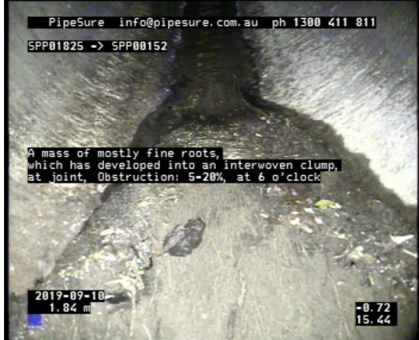
Photo: 1_3A, Media No:: 100919_1, 00:00:57 1.84m, A mass of mostly fine roots, which has developed into an interwoven clump, at joint, Obstruction: 5-20%, at 6 o'clock
