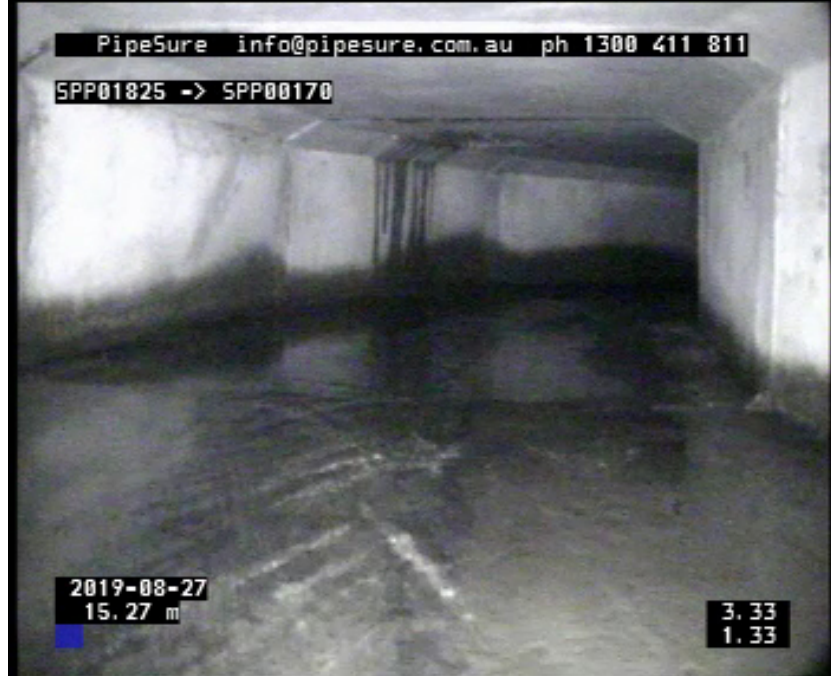
Photo: 4_3A, Media No:: 280819_1, 00:05:03 17.58m, The conduit curves to the right, length: 1000 mm
