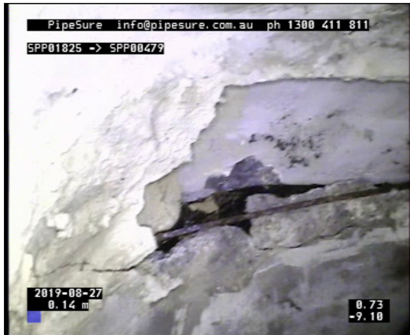
Photo: 3_3A, Media No:: 280819_1, 00:08:37 0.14m, Steel reinforcement is visible and projecting into the conduit, at joint , from 10 to 2 o'clock
