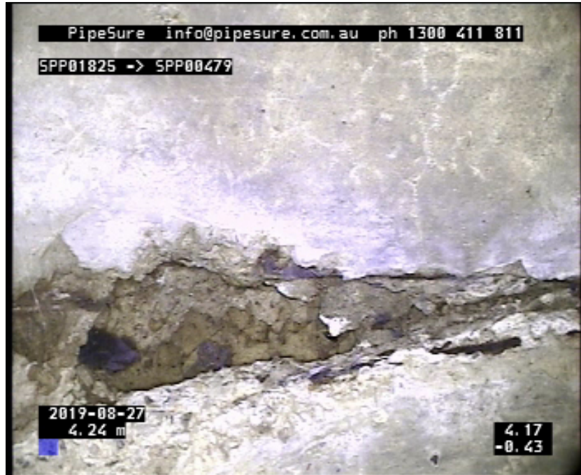
Photo: 3_6A, Media No:: 280819_1, 00:02:53 4.24m, Joint displaced angular, angular displacement 10 °, at 11 o'clock
