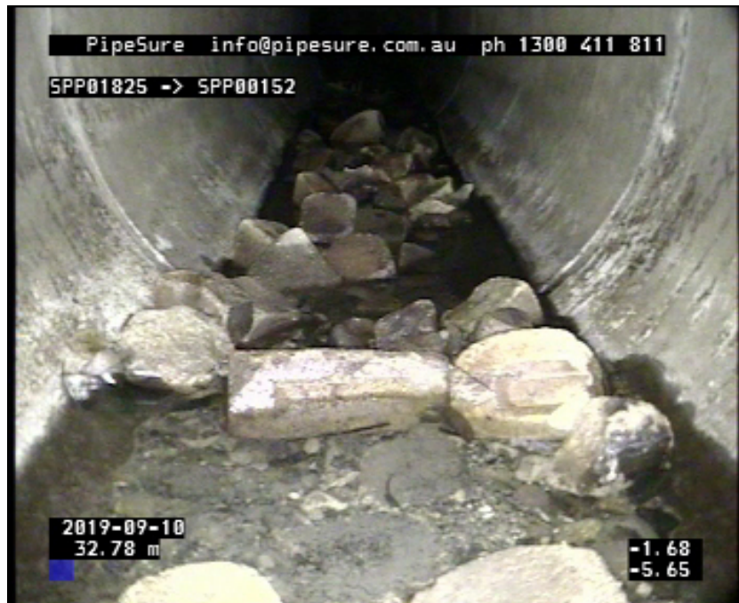
Photo: 1_15A, Media No:: 100919_1, 00:11:33 32.78m, Deposits in the invert, gravel or rubble, Obstruction: 5-20%, from 4 o'clock, to 7 o'clock, large rubble in the invert obstructing / large rubble in the invert obstructing
