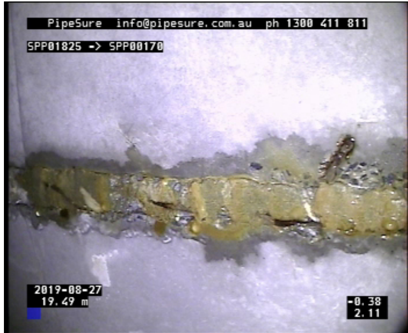
Photo: 4_4A, Media No:: 280819_1, 00:05:40 19.49m, Infiltration, sweating--slow ingress of water, no visible drips, from 12 o'clock, to 12 o'clock, at the joint<less then 5% / at the joint<less then 5%
