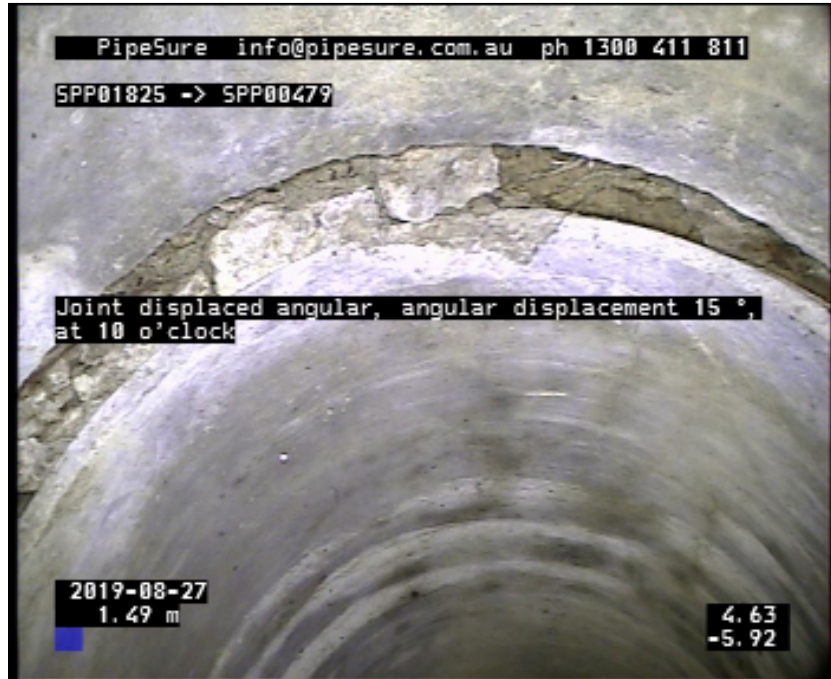
Photo: 3_4A, Media No:: 280819_1, 00:01:38 1.49m, Joint displaced angular, angular displacement 15 °, at 10 o'clock
